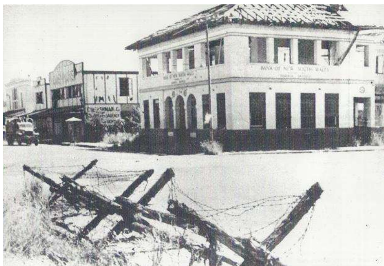
Bank of New South Wales in WWII, Smith Street, Darwin, from a postcard. The building is now the Westpac Bank at the southern end of the Darwin Mall. (Peter Farnden)
