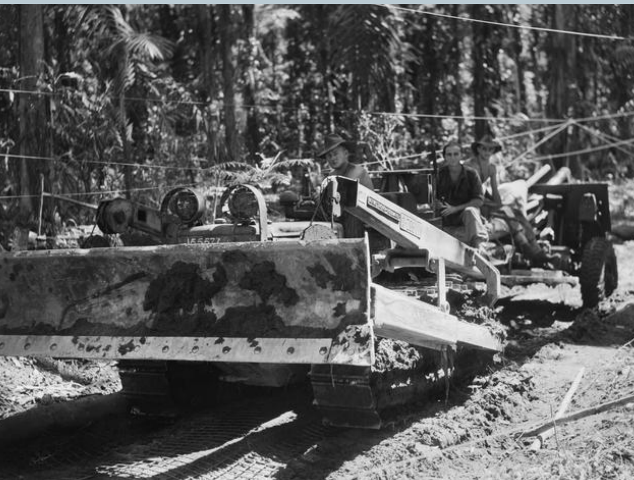
Troops of the 2nd Field Regiment use a bulldozer to tow a 25-pounder along the corduroyed Buin Road, 25 May 1945.
