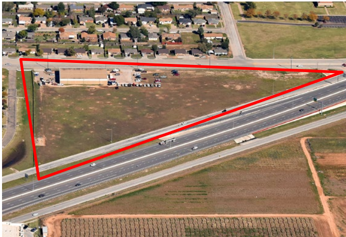
Building Site on TTU campus NW Corner – Erskine and Loop
